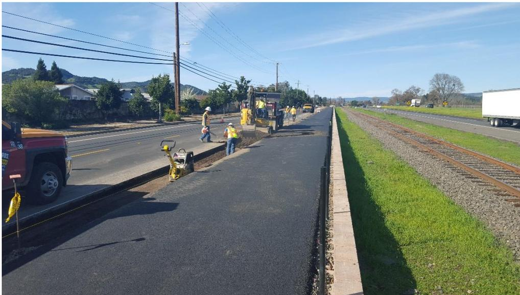
GBI grading and compacting aggregate base at bike path
